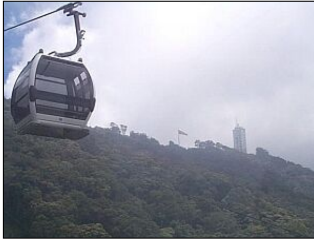
The cable car and Humboldt hotel represent a potential threat for the conservation of the park.
