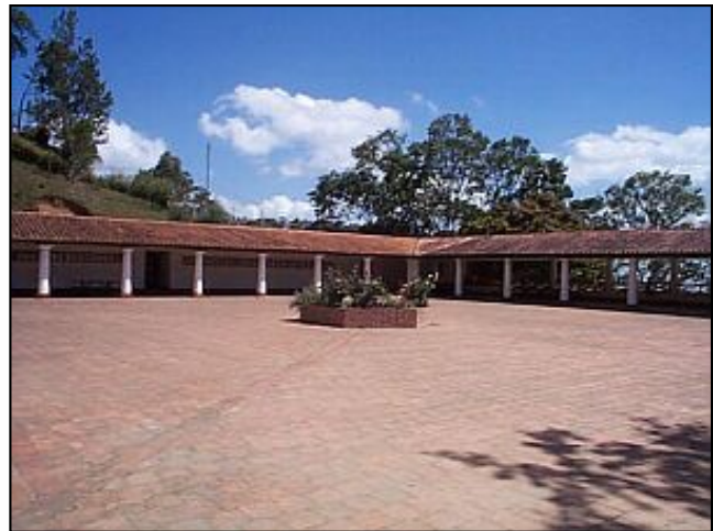
Photographs of the Los Venados information center. The numerous signs and the excellent condition of the buildings contrasts with the neglected north side of the park.
